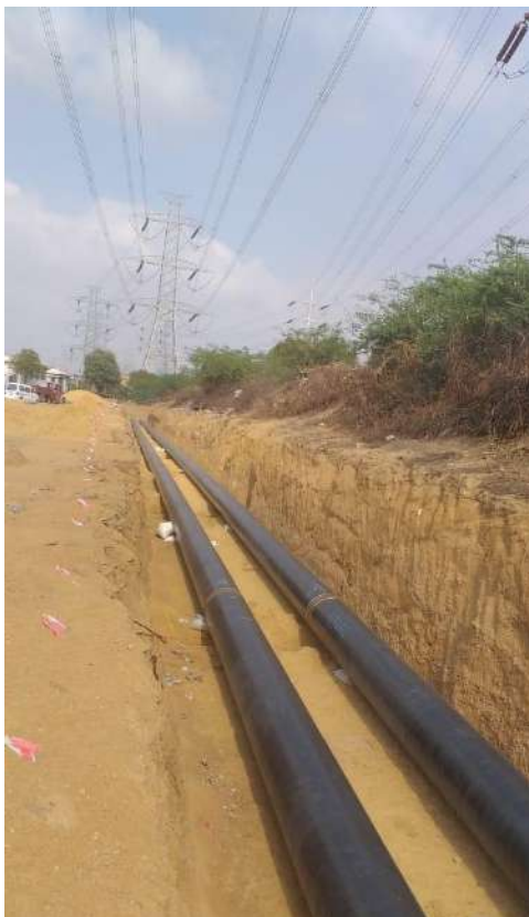
PSO - Development of pipeline link between PSO Booster Station and White Oil Terminal Station PARCO. 24 inch dia pipeline
