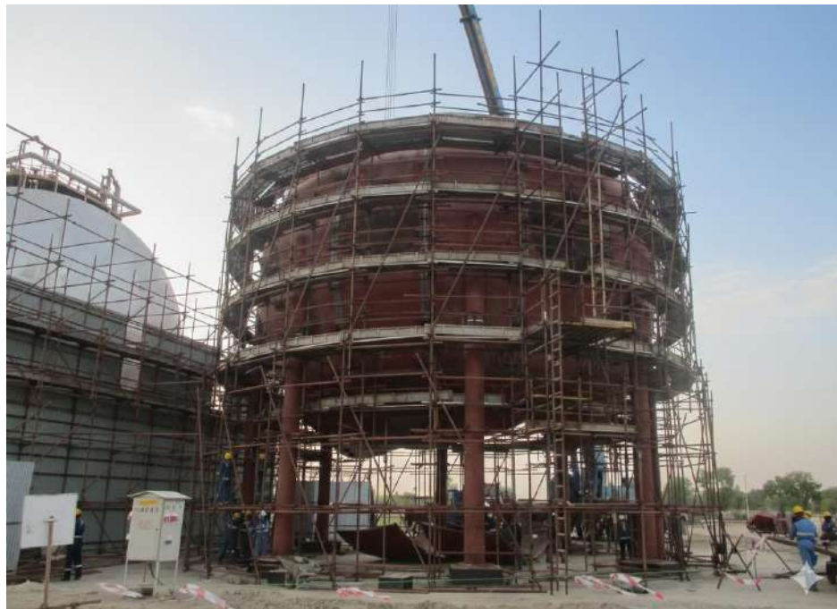
PARCO – New LPG Sphere of Capacity 1530 M3 at PARCO Mahmood kot Refinery - ATL / CIMC Honto (China)
