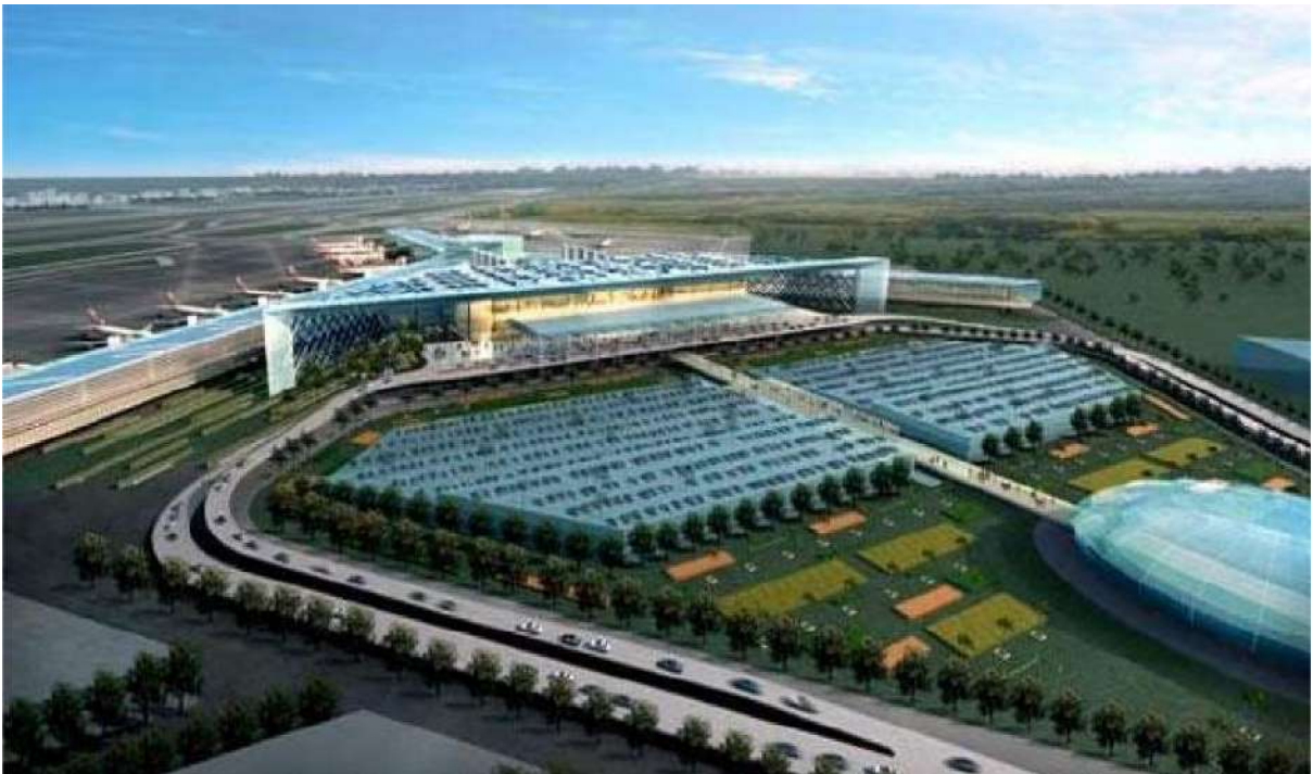
CAA – New Islamabad International Airport Fuel Hydrent Refuling System
