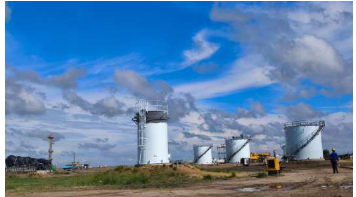
PPL - Rehabilitation of Field Storage Tanks at Zafir Gas Processing facility Project (09 Nos. Tank)
